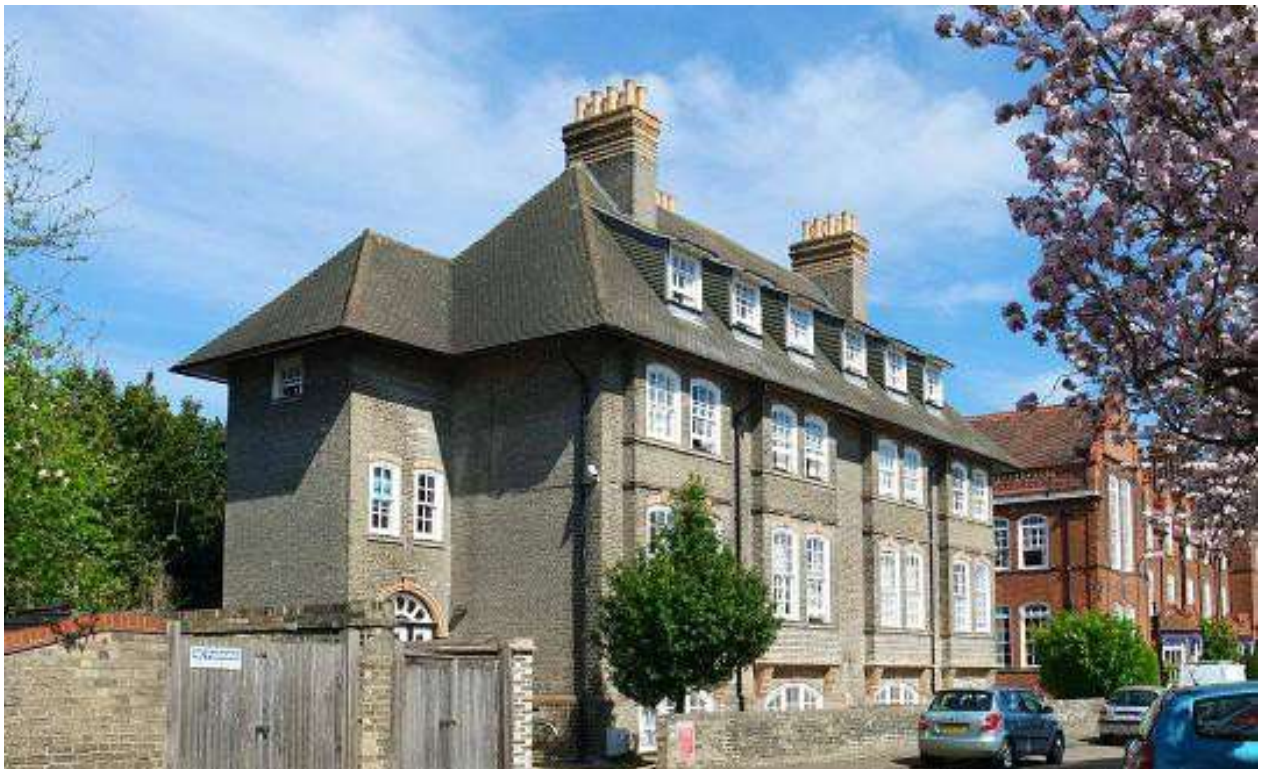
Wollaston Lodge's west front, view from the drive
