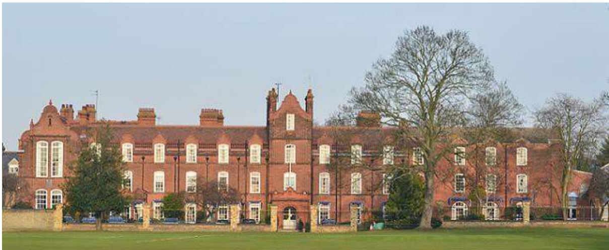
Wileman Building's west front, view from Gresham Court
